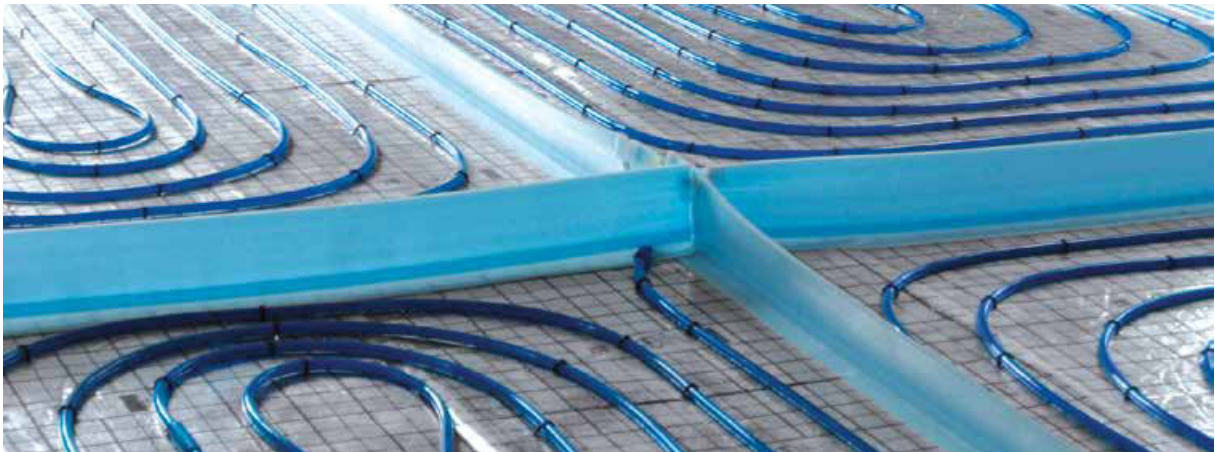
Fig. 14. Distribution of heating fields with dilatation gaps
