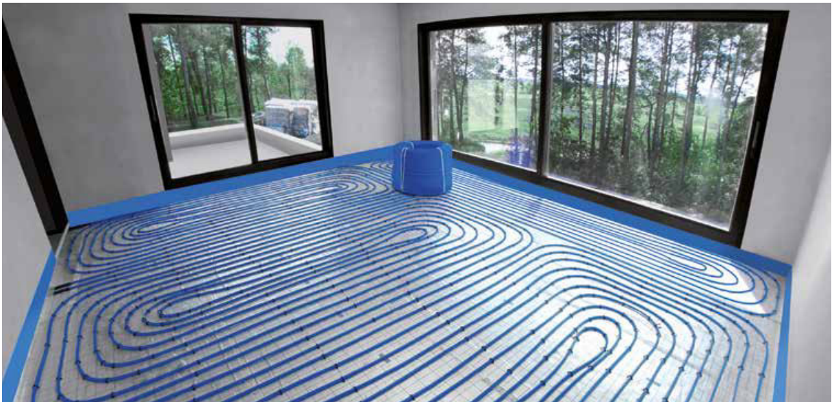
Fig. 3. Floor heating installation in single-family building, employing bluePERT pipes and KAN-therm Tacker system.
