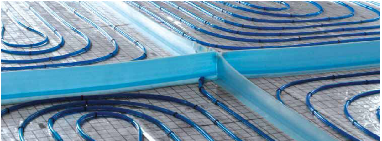
Fig. 14. Distribution of heating fields with dilatation gaps
