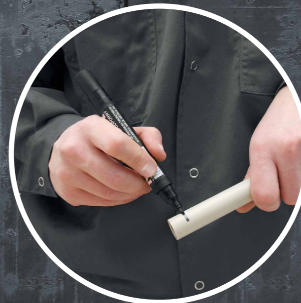
03 Marking the welding depth.
