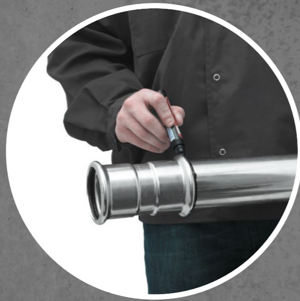
05 Marking the required insertion depth of the pipe into the fitting - essential for achieving the right connection strength.
