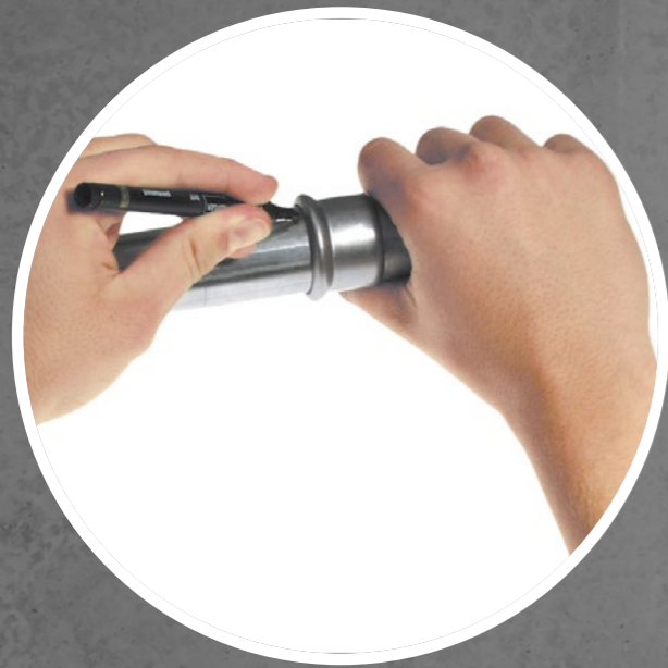
05 Marking the required insertion depth of the pipe into the fitting - essential for achieving the right connection strength.
