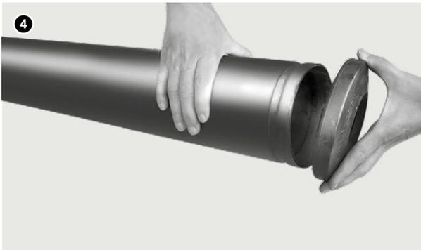
**4. First, install the gasket on the larger pipe**
