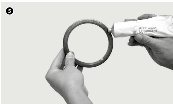
**5. Check the gasket grade and lubricate it**
